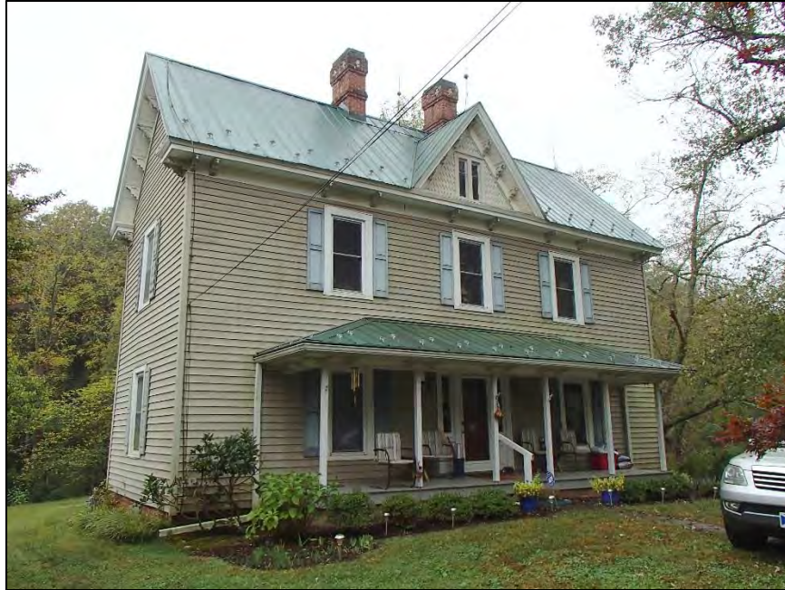
Figure 6: Charlie Dobbins House, north elevation
