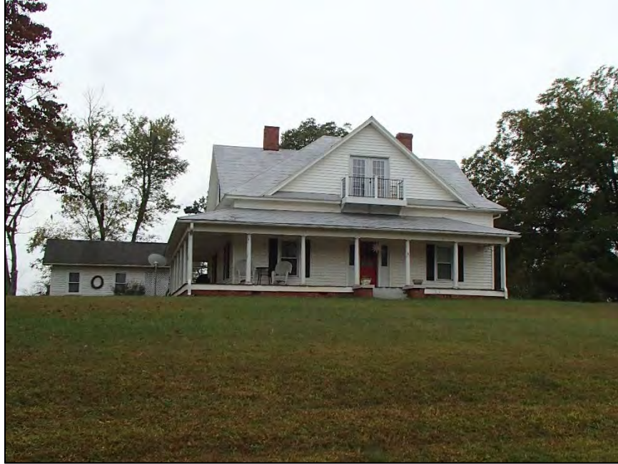
Figure 64: Riley Faulk House (SR 179) at 1218 Quaker Church Road, with vinyl siding, added balcony, and replacement windows
