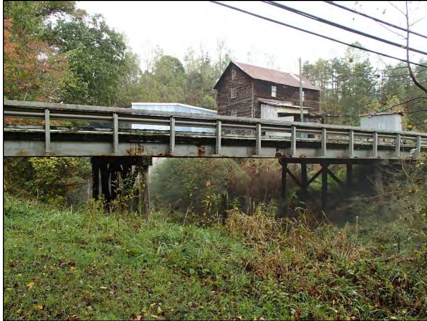
Figure 8: Bridge 12, south elevation
