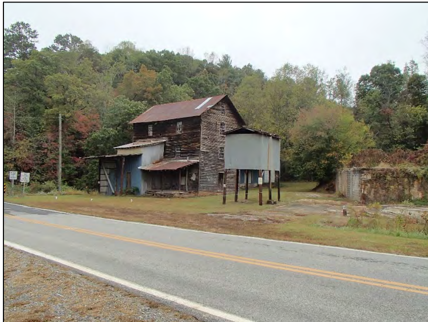
Figure 5: Dobbins Mill, southeast corner
