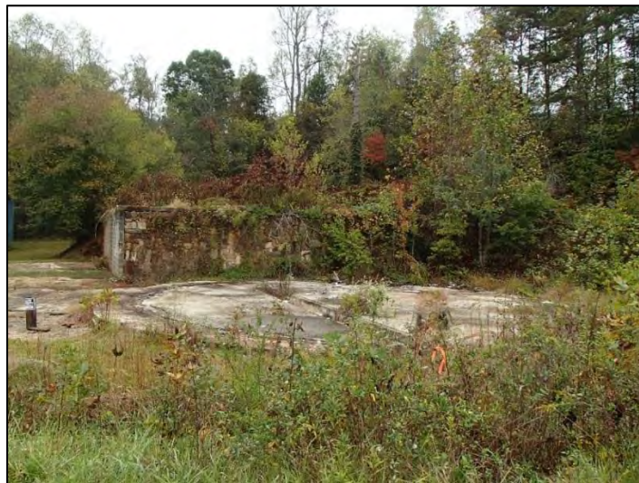
Figure 22: Dobbins Mill, grain bin foundation with retaining wall in background
