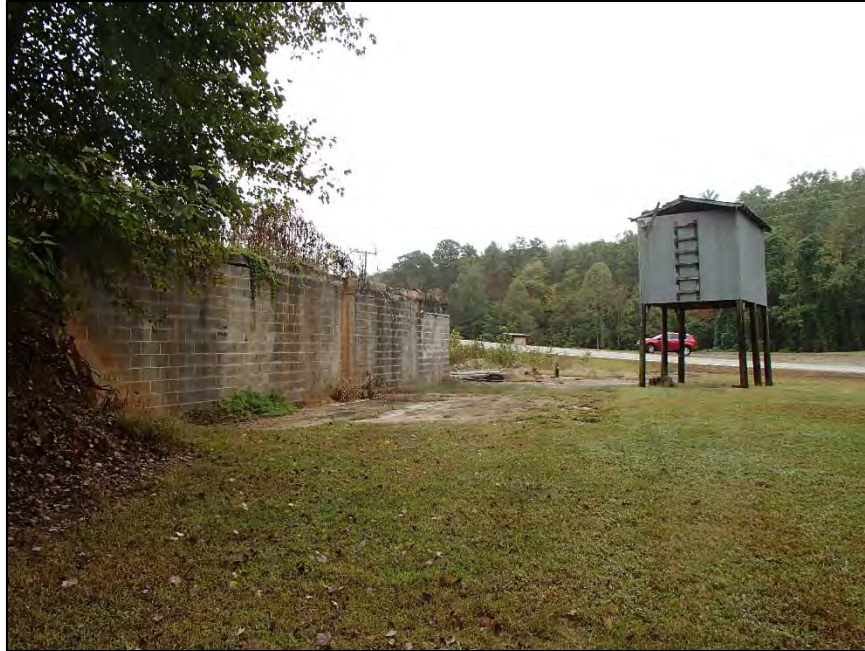
Figure 25: Dobbins Mill, facing southeast toward loading dock and retaining wall
