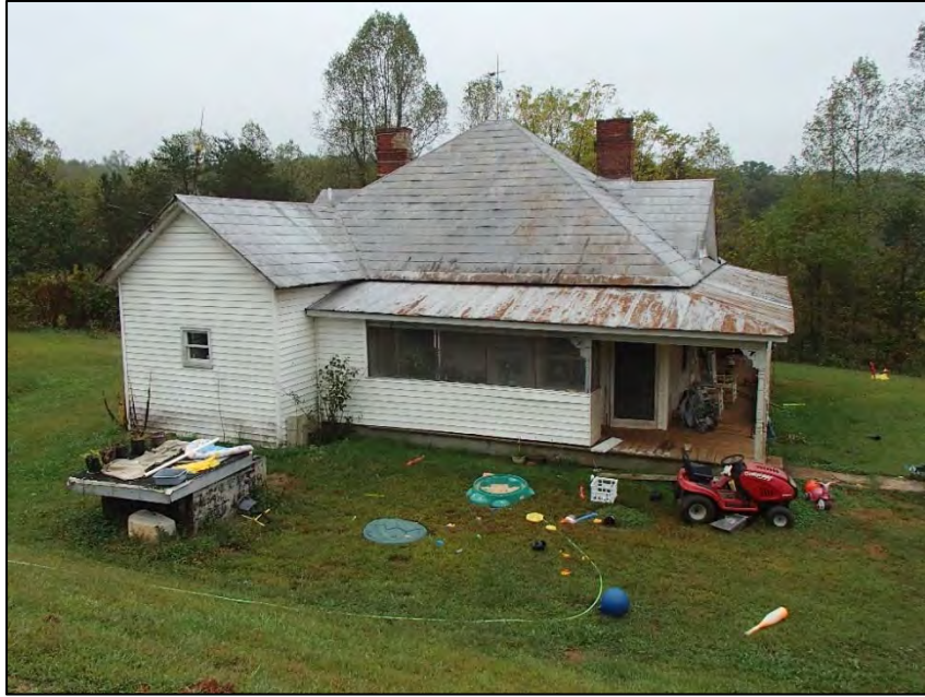
Figure 57: Dobbins House, north elevation
