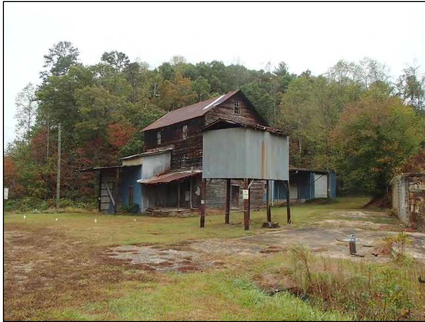
Figure 21: Dobbins Mill, loading dock and in-ground scales
