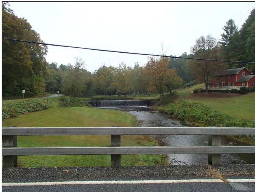
Figure 11: Dam at Kapp's Mill. The house in the image is a heavily remodeled store. This view is facing north toward the mill dam. Kapp's Mill is located to the east, just out of the frame. The bungalow is located to the west, and the miller's house to the south.
