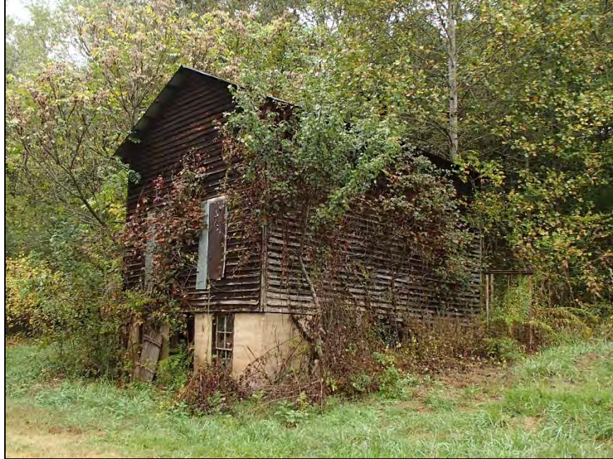
Figure 43: Charlie Dobbins House, tobacco packhouse, southeast corner
