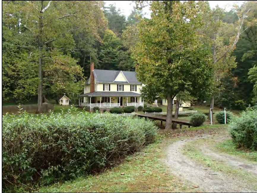
Figure 10: Kapp House at Kapp's Mill
