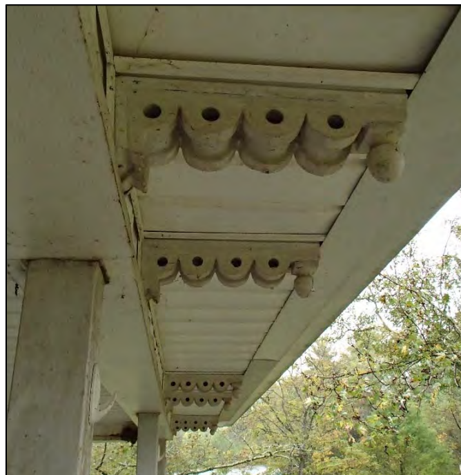
Figure 33: Charlie Dobbins House, porch eave detail
