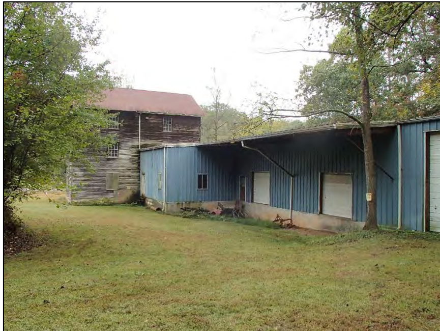
Figure 16: Dobbins Mill, north elevation and addition
