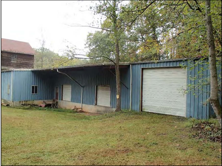
Figure 19: Dobbins Mill, east elevation of rear addition
