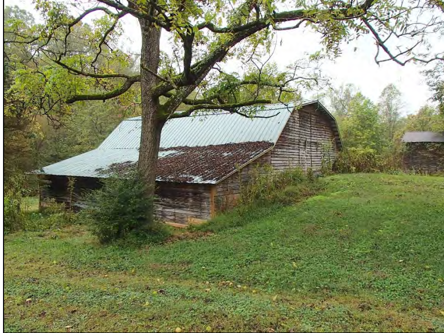
Figure 41: Charlie Dobbins House, barn, northeast corner
