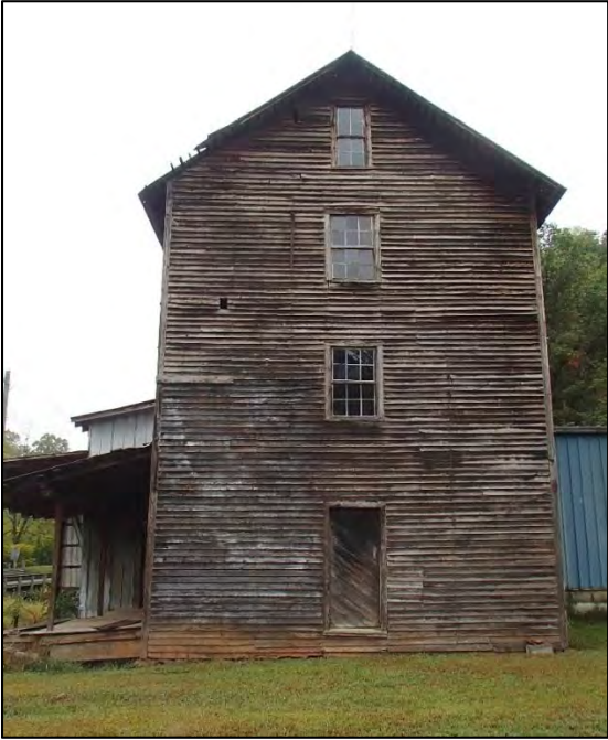
Figure 14: Dobbins Mill, east elevation
