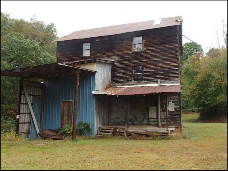
Figure 13: Dobbins Mill, south elevation
