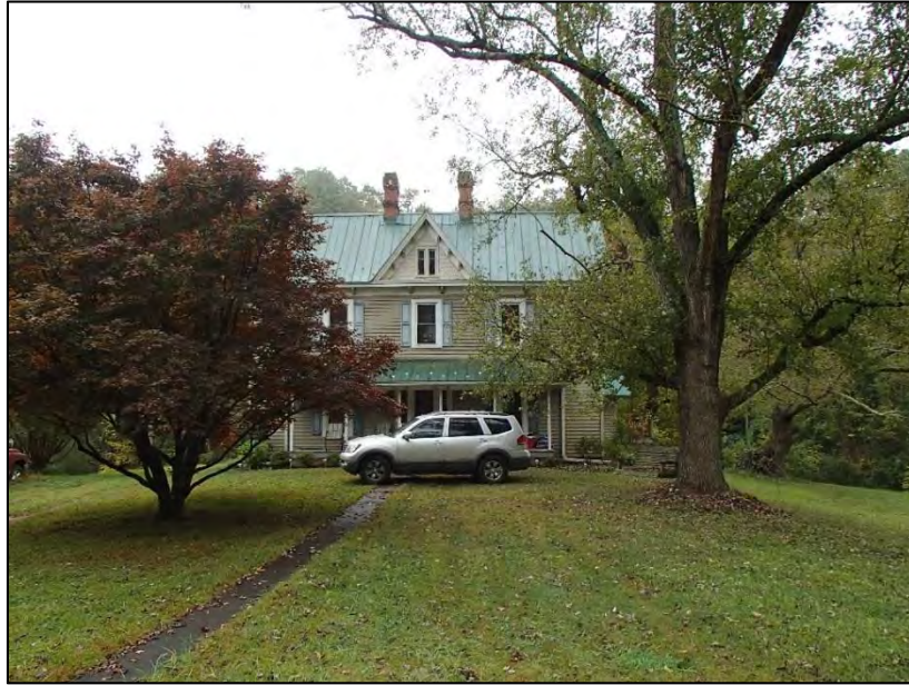
Figure 32: Charlie Dobbins House, north elevation
