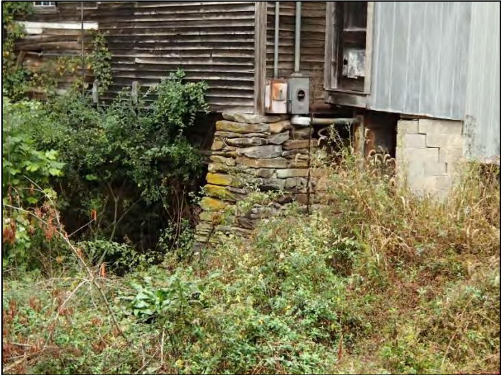
Figure 18: Dobbins Mill, stone foundation pier
