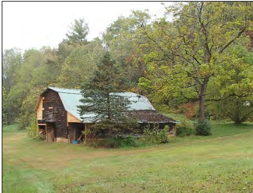
Figure 40: Charlie Dobbins House, barn, southeast corner
