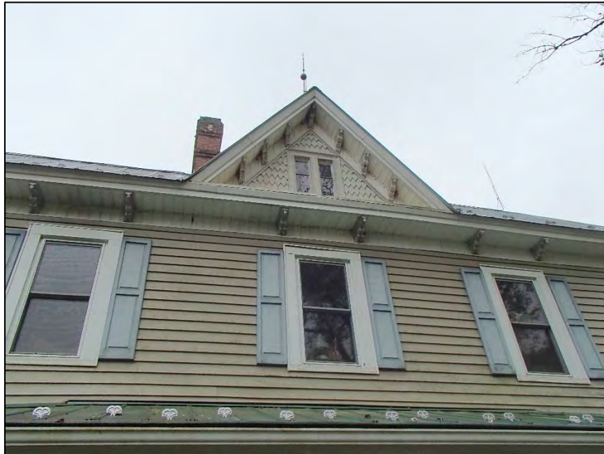
Figure 35: Charlie Dobbins House, roof gable and eave
