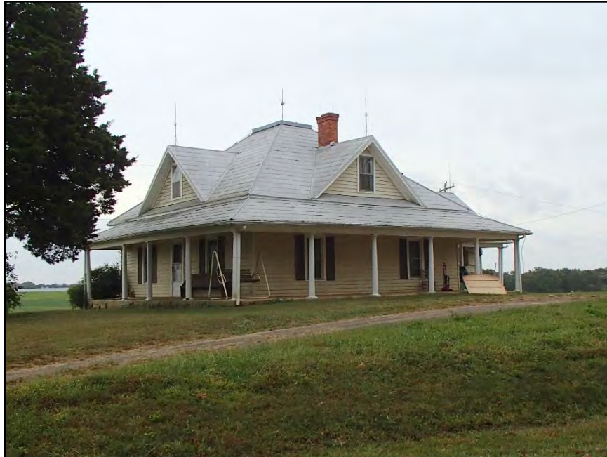
Figure 63: Unsurveyed House at approximately 182 Miller Gap Road, close to Music Lane, with vinyl siding, original windows, and original shingles
