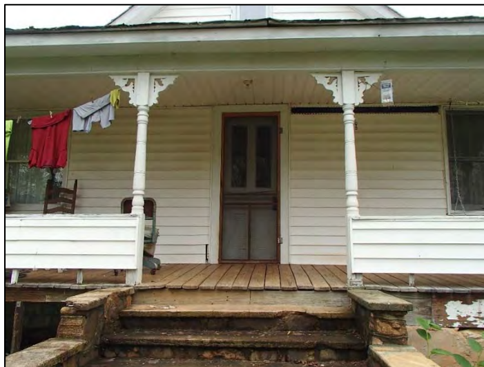
Figure 54: Cleveland Dobbins House, south elevation detail
