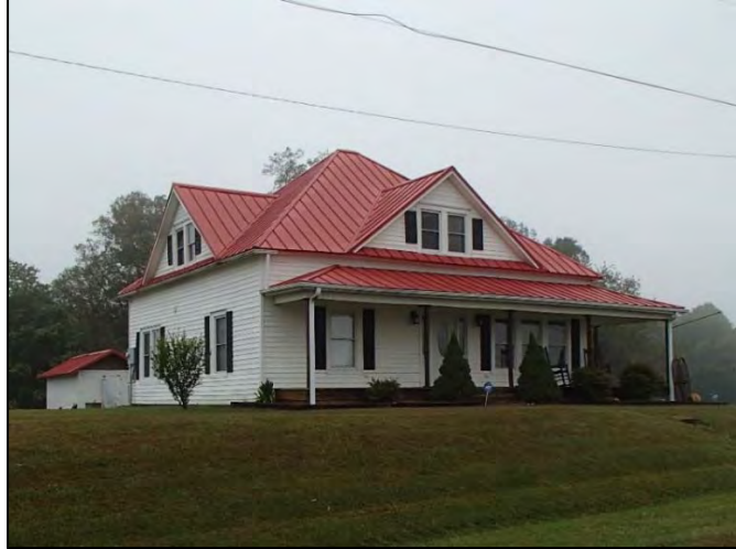
Figure 62: Unsurveyed house at 241 Judsville School Road, with vinyl siding, replacement windows, new porch and roof materials, missing chimneys
