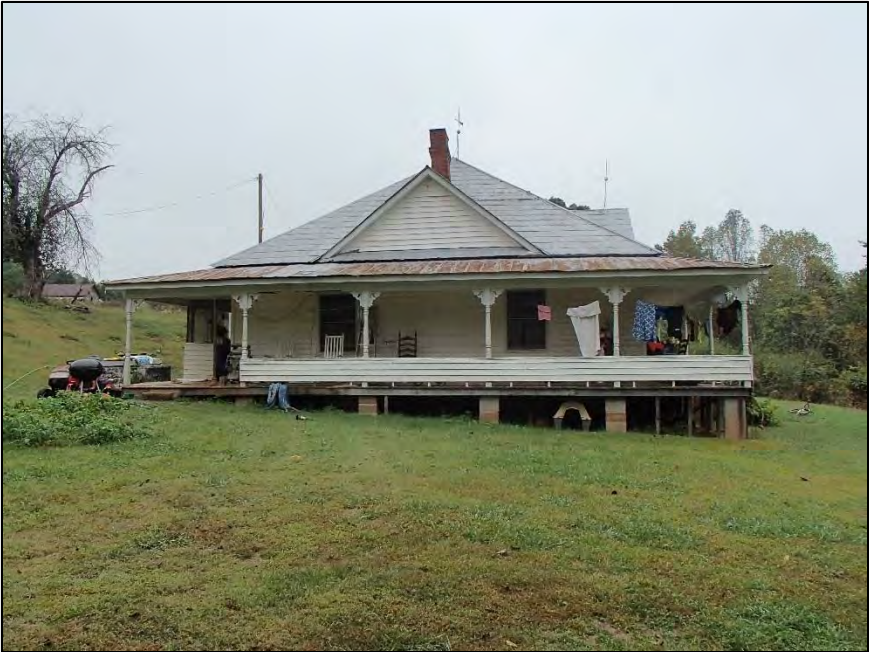
Figure 55: Cleveland Dobbins House, west elevation
